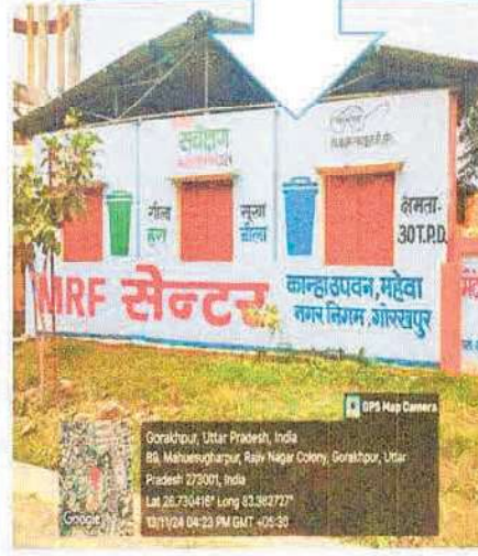
Material Recovery Facility Mahewa
